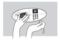
3. Cut the ceiling drywall along the mark you made in Step 2 to create the mounting opening.
